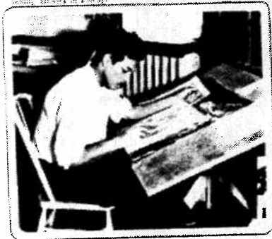
MIGUEL ALFERREZ, A TALENTED MEXICAN WOOD CARVER, is busy working on the symbolic statues for the side water cars and doors of the new Palmolive Building, each symbol representing some primitive woman preserved for "schoolgirl complexion." The cars of high speed, fully automatic elevators, however, are probably the finest and water installations ever made in an American office building.
